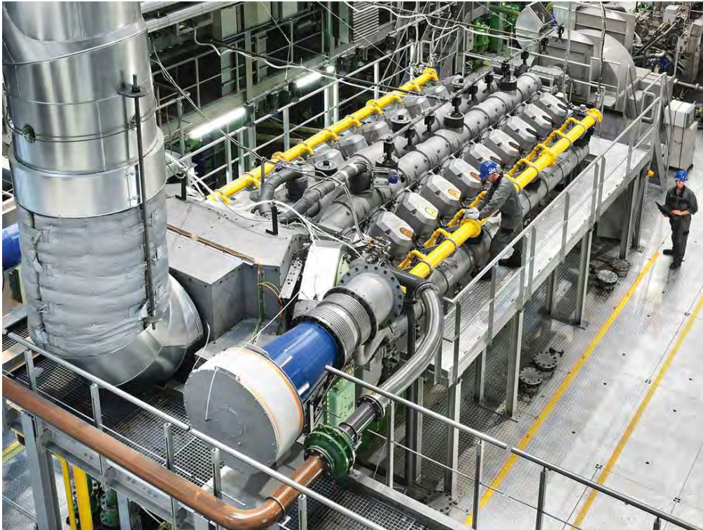
Fig. 18: MAN's "H2-ready" gas engine (source: https://www.man-es.com/de/unternehmen/pressemittelungen/pres-details/2021/11/04/h2-ready-man-gas-engines-make-hydrogen-use-in-power-plants-possible )
