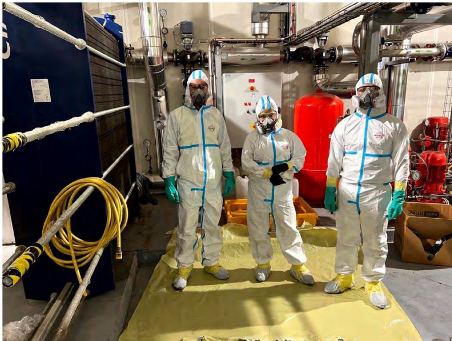
Fig.87: Full protective clothing before starting the deinstallation and decontamination work
