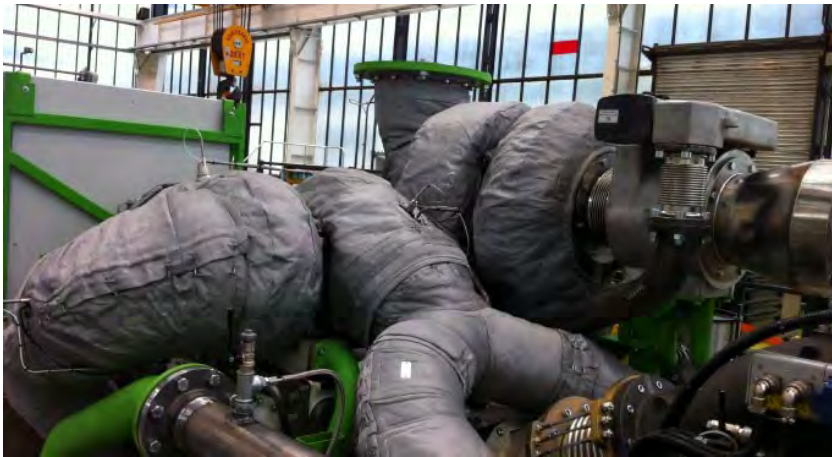
Fig12: Motor insulation with insulating mats
