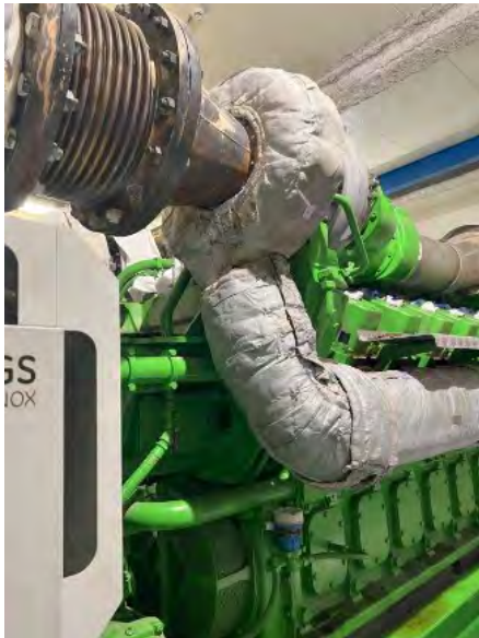
Fig.1: Thermally insulated gas engineFig.
